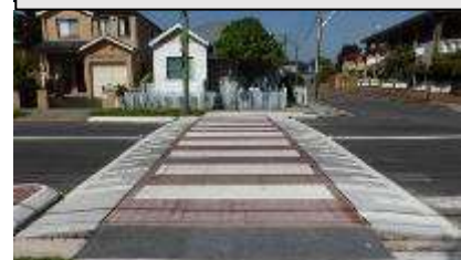
Raised Pedestrian Crossing
