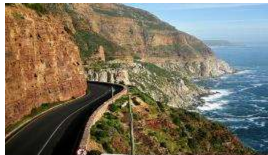
Stone Masonry barrier on Chapmans Peak Drive
