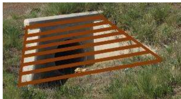
Safety treatment for cross-drainage culverts will prevent errant vehicles from getting damaged by the structures
