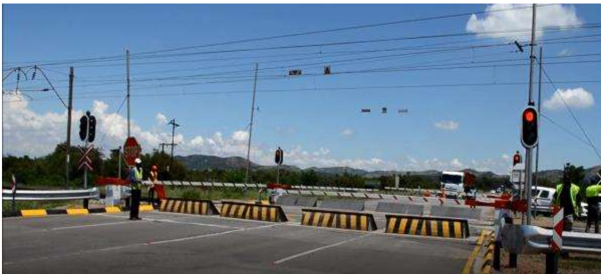
Figure 36: Boschhoek Railway Level Crossing with Barriers
