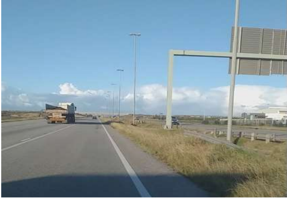
Figure 5: Short Barrier Section – Length of Barrier Insufficient and Very Narrow Working Width to Lamp Post
