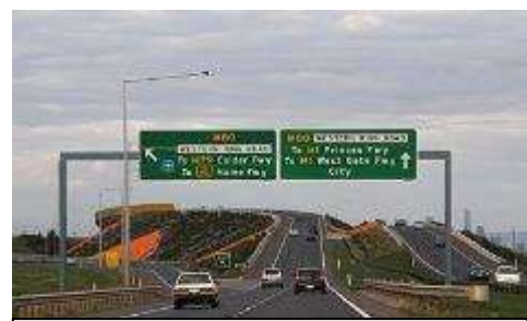
Example of protected gantry
