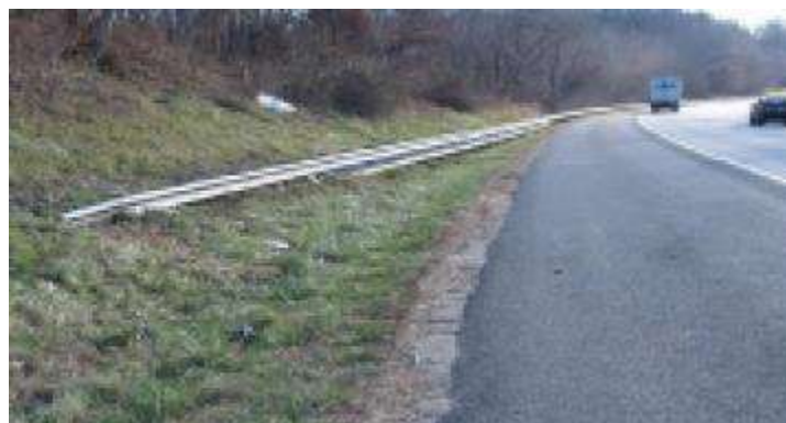
Figure 20: Buried in Backslope Barrier Terminal
