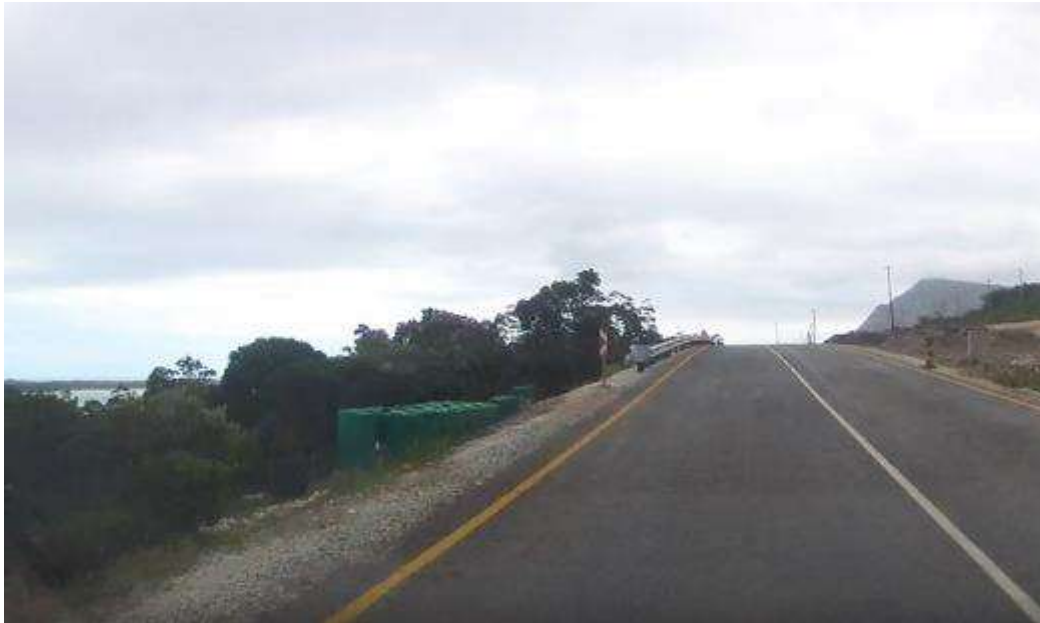
Figure 8: Illustration of Inadequate Working Width and Length of Need
