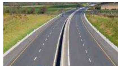
Well maintained horizontal curve
