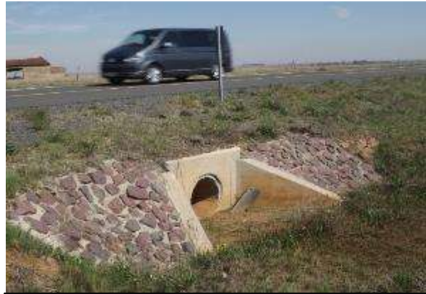
Drainage structure close to road
