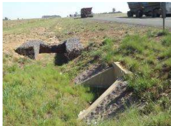
Inlet structures within clear zone
