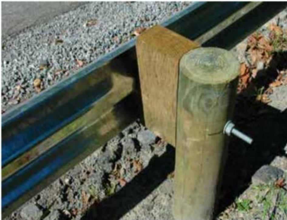
Figure 15: Illustration of Post and Beam Connection
