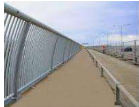
Protected pedestrian walkway
