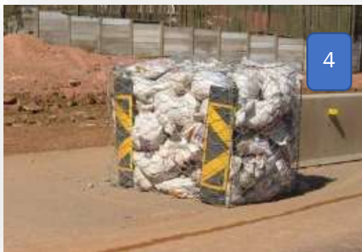
1 Violating Zone of Intrusion 2, 3 & 4 No energy absorbing crash cushion or transition
