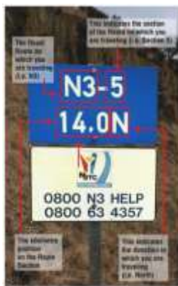
Figure 4-1: Typical kilometre marker with explanations
