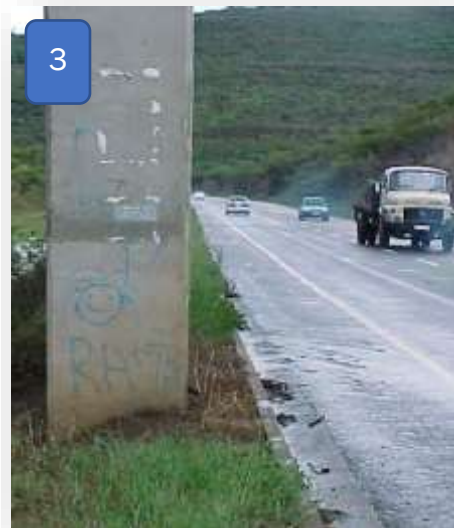
1 Violating Zone of Intrusion 2, 3 & 4 No energy absorbing crash cushion or transition
