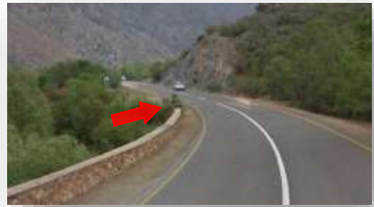
Hidden access on inside curve
